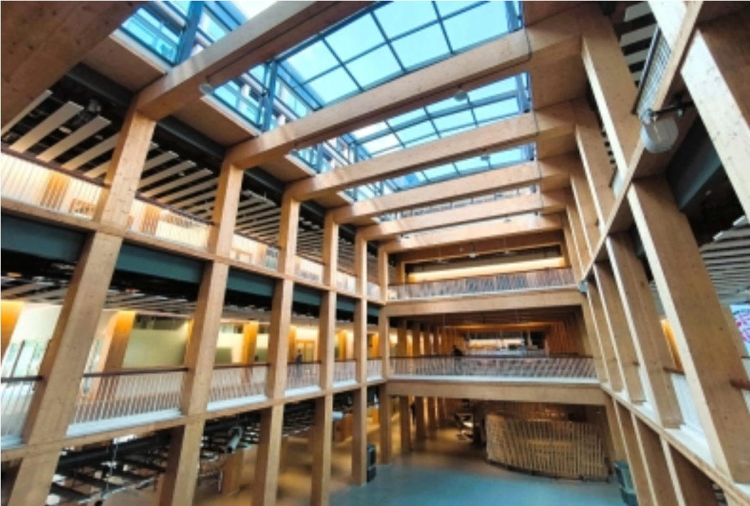
The interior of Gaia and its skylight. Associate professor Tham Kwok Wai, an expert in Indoor Air Quality, and associate professor Shinya Okuda, an award-winning architect specialising in timber, both assessed Gaia and confirmed that the timber itself did not cause the mould growth. They identified that condensation and rain were the primary factors, a statement issued by NTU said yesterday. — Picture courtesy of NTU Singapore
